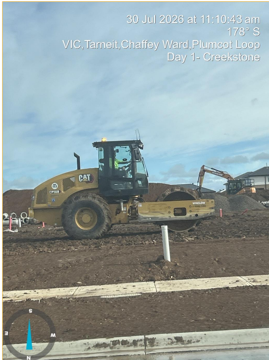
Figure 3: Fill Compaction (Source: C&amp;T)
