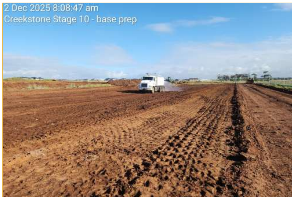
Figure 3: Moisture Conditioning Subgrade Prior to Fill Placement (Source: C&T)
