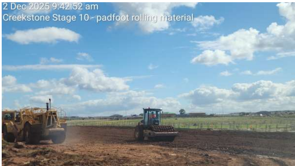
Figure 6: Fill Compaction (Source: C&T)
