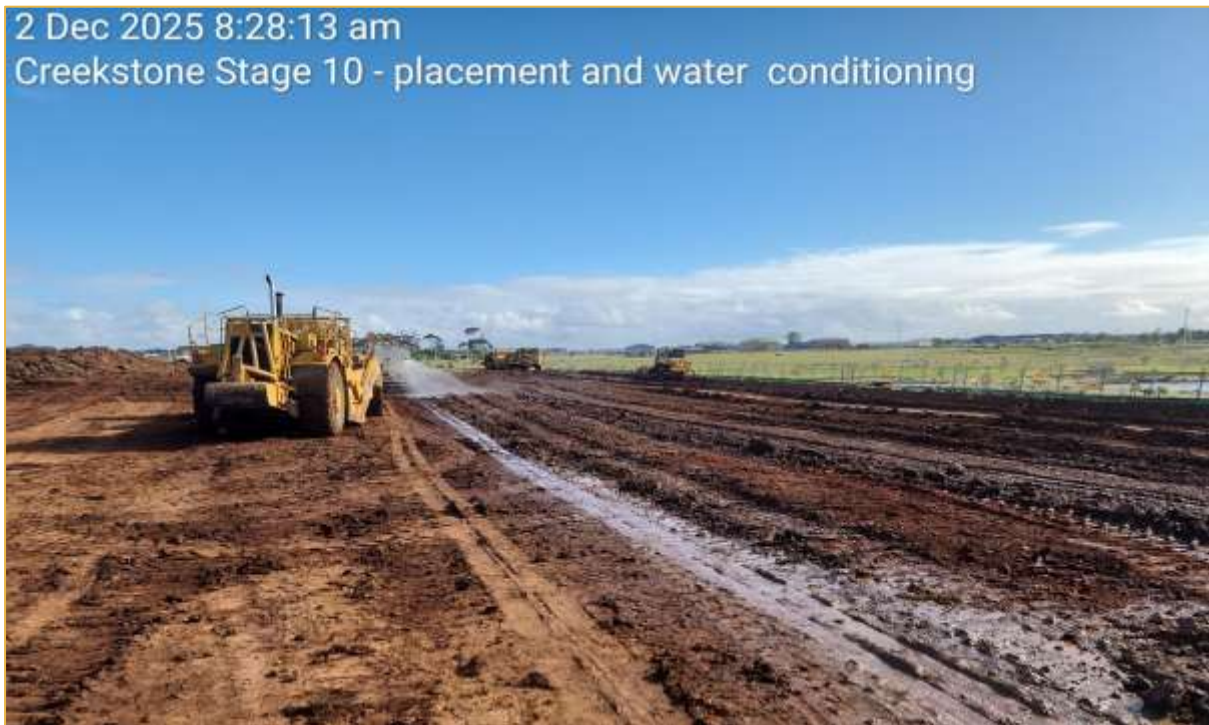
Figure 5: Spreading of Fill Material & Moisture Conditioning (Source: C&T)
