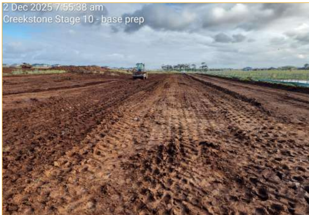
Figure 2: Subgrade Preparation (Source: C&T)
