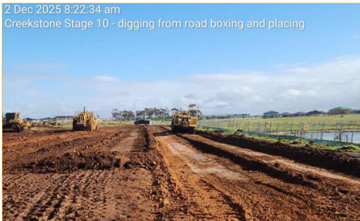
Figure 4: Spreading of Fill Material Across the Placement Zones (Source: C&T)
