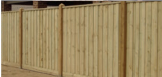
Capped timber palings with exposed posts
