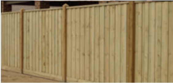
Capped timber palings with exposed post
